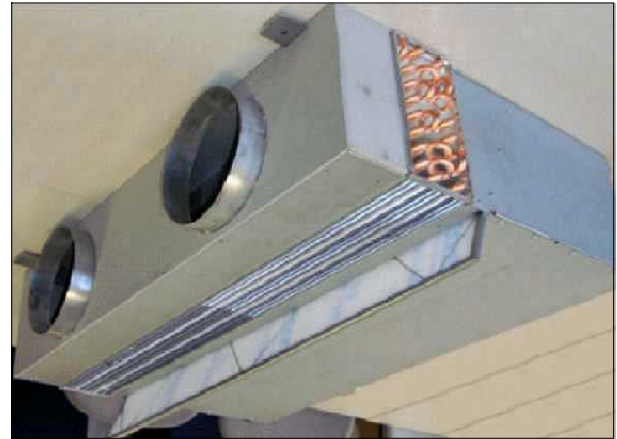
2. Replacement of plug-in filter
