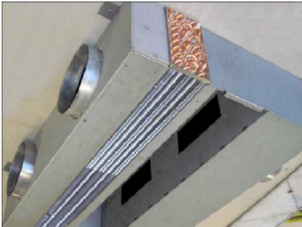
3. Removal of lower plate, vacuum-cleaning of heat exchanger on the pressure side
